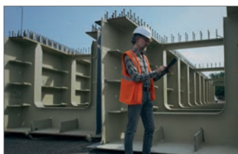
STAHLBAU STEEL CONSTRUCTION
